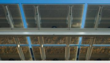
Backrails are glued onto the reverse side of the modules and these are inserted into the carrierrails of the substructure. The Backrails are hooked into the Carrierrails with the aid of gravity.
